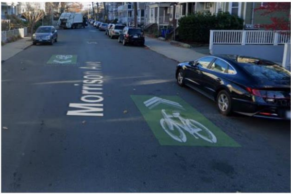
Shared Lane Marking with Green Box
