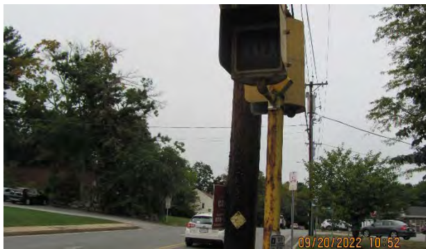
Figure 10. Older pedestrian signal heads do not provide a countdown timer on some corners of the intersection. Some push buttons need updating too.
