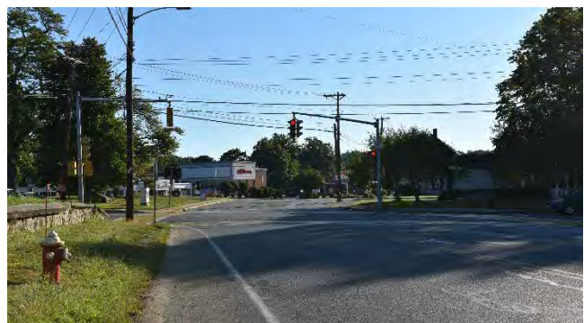
Figure 9. Lakeview Avenue eastbound approach provides only two signal heads for three travel lanes.
