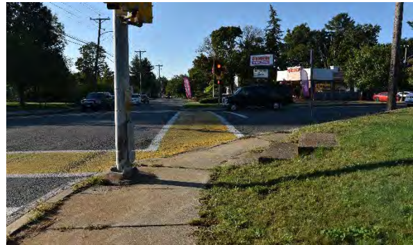
Figure 13. Lack of drainage options at a low point in the northwest corner of the intersection.
