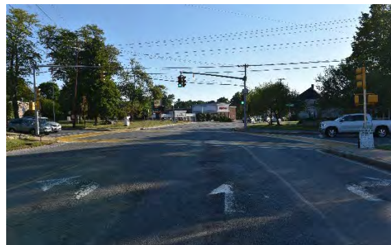
Figure 5. Lakeview Avenue eastbound approach. Significant difference in width between approach and departure lane. Worn pavement markings.
