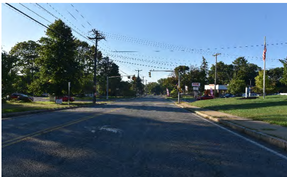
Figure 6. Worn pavement markings on Mammoth Road southbound approach to Lakeview Avenue. Including pavement rutting in southbound lanes.
